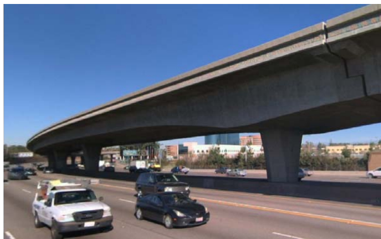
I-5 Highway Viaduct – Santa Ana
